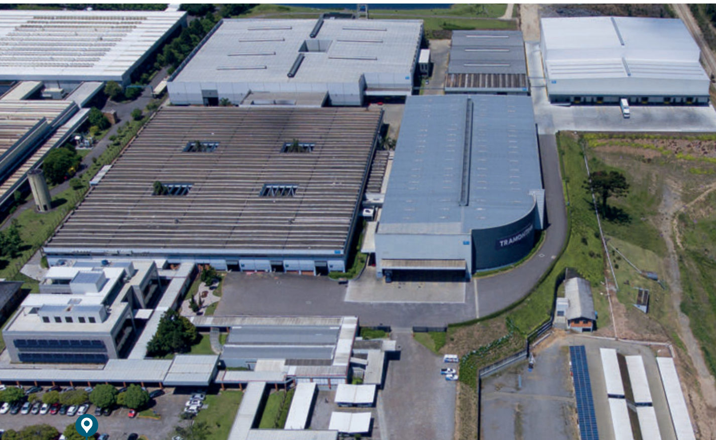
ELETRIK Manufacturing Facility | Fábrica ELETRIK
